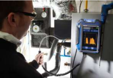
Fig. 45: Spillage test: Searching for condensate
