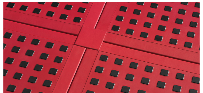
Final Expansion Joint Installation
