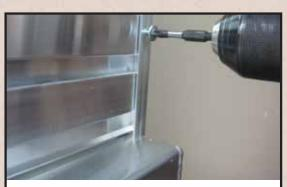
11. Attach LONG SIDE MOLDINGS (E) to the edges of SLATWALL PANELS. Install a DRILL POINT PHILLIPS SCREW (f) on each MOLDING in the location shown (back).
