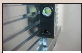
10. Check slatwall face for vertical and tighten HEX BOLTS and NUTS on UPRIGHTS.
