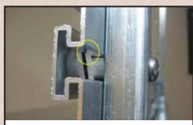
8. Rotate first SLATWALL PANEL up onto the two lowest ALUMINUN NUTS. Tighten SCREWS just enough to keep ALUMINUM NUTS engaged in SLATWALL PANEL.
