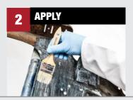
Apply 2 – 3 light coats of **Rust Seal** 5 – 10 minutes apart. Do not apply to sand blasted or painted areas. Allow to dry fully. **Rust Seal** does not require a top coat unless exposed to outdoor conditions. Body filler and top coat can be used after **Rust Seal** has fully dried.
