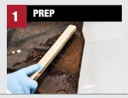
Remove loose scale with a wire brush. Clean with **SEM Solve** to remove oil, grease and dirt. Blow off with compressed air.
