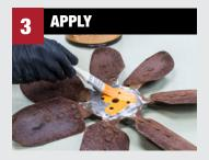
Apply 2 – 3 medium wet coats of **Rust Shield** with a brush or spray gun allowing a 3 – 5 minute flash time between coats. Maximum rust protection is achieved from thicker applications. Allow final coat to cure 24 – 48 hours before returning part to service.
