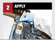
Apply 2 – 3 light coats of **Rust Seal** 5 – 10 minutes apart. Do not apply to sand blasted or painted areas. Allow to dry fully. **Rust Seal** does not require a top coat unless exposed to outdoor conditions. Body filler and top coat can be used after **Rust Seal** has fully dried.
