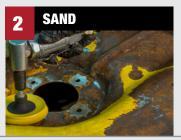
Remove loose rust scale by sanding, grinding or using a wire brush.
