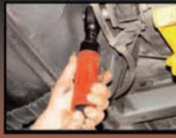
2001 Lexus RX300 Rear Trailing Arm ASE Lexus Master Technician, Bob, Springfield, MO
