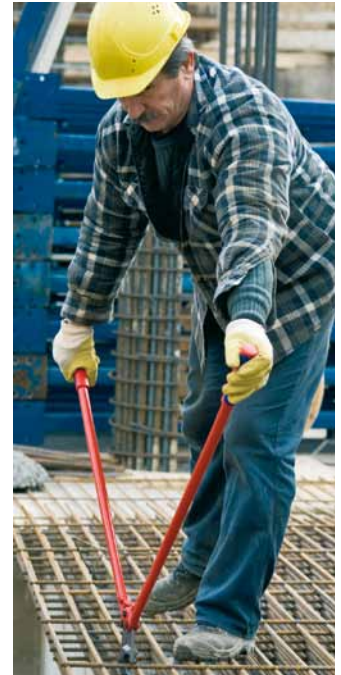
The special shape of the mesh cutter head enables it to cut structural steel that is lying down flat
