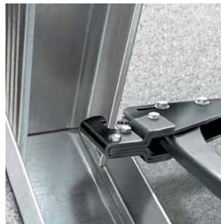
Preparing the pliers for connection of two metal section sheets
