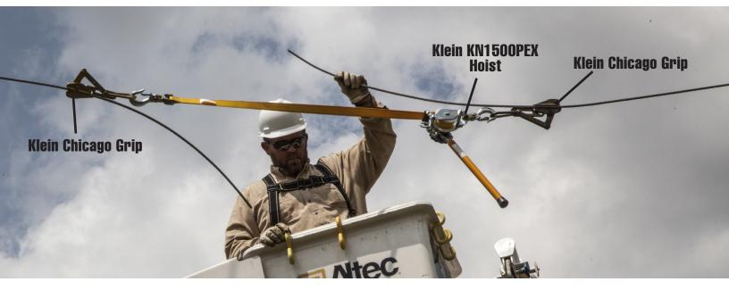
2. Connect the KN1500PEX Web Strap Ratchet Hoist to each grip, and ratchet to the desired tension to make the splice.
