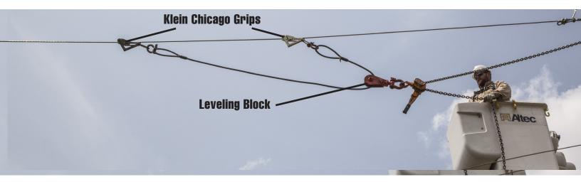
Ratchet the chain hoist to the desired tension, as shown in the picture below.
