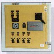
To insure quality our control systems offer output regulators for temperature control. Heat is divided into 4 zones for economical operation.
