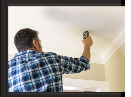
Using moisture meters to precisely measure penetration levels during the repair and drying process assures that damaged areas are properly repaired and reinforced. Effectively structural drying is a process in itself and moisture meters can also measure the progress of repairs and help to identify and eliminate trapped moisture.
