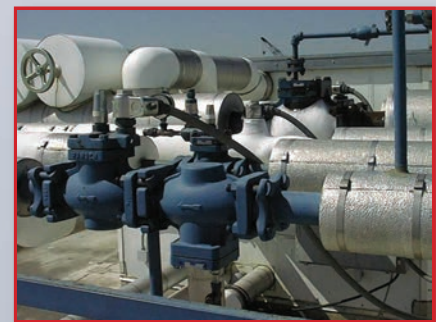
Maintaining ammonia refrigeration piping
