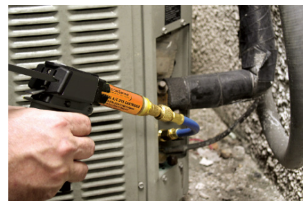
Step 3: Inject, then discard empty cartridge.
