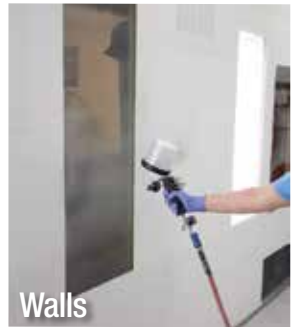
Walls Apply 3M™ Booth Coating on walls.
