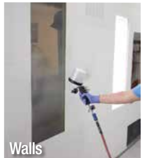
Walls Apply 3M™ Booth Coating on walls.
