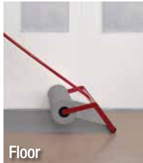
Floor Apply 3M™ Dirt Trap Protection on floor.
